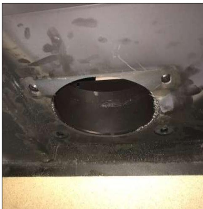
Note: The lid can be removed for easy viewing and spigot change over. Once the lid is placed back on the stove, use blanking plate supplied to cover the hole left in the lid for the top outlet spigot.
